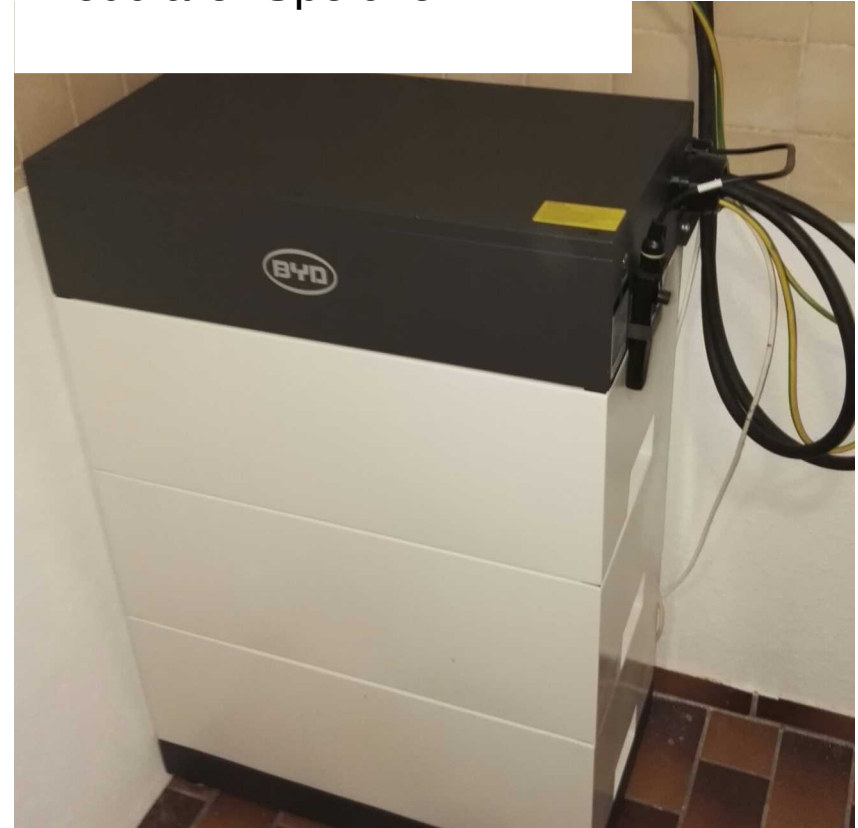
BYD 10,5 kWh 51.2V LFP [LiFePo]
